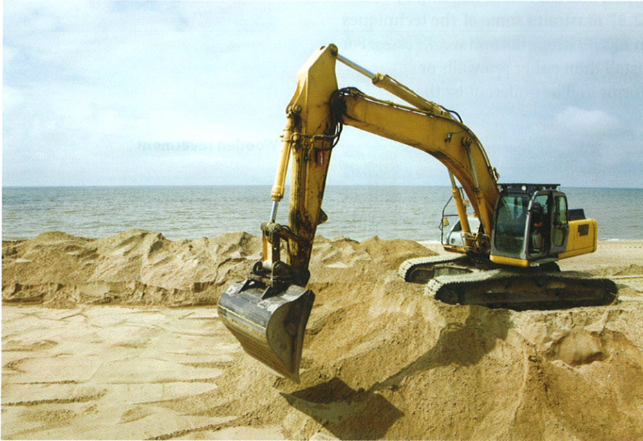
Figure 2.38: Beach replenishment in progress
