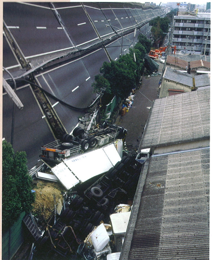
Figure 3.25: Some of the earthquake destruction
